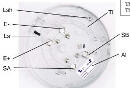
The detector is plugged in the analog base 3312. The COM loop / Ext. LED are connected to the analog base 3312.
